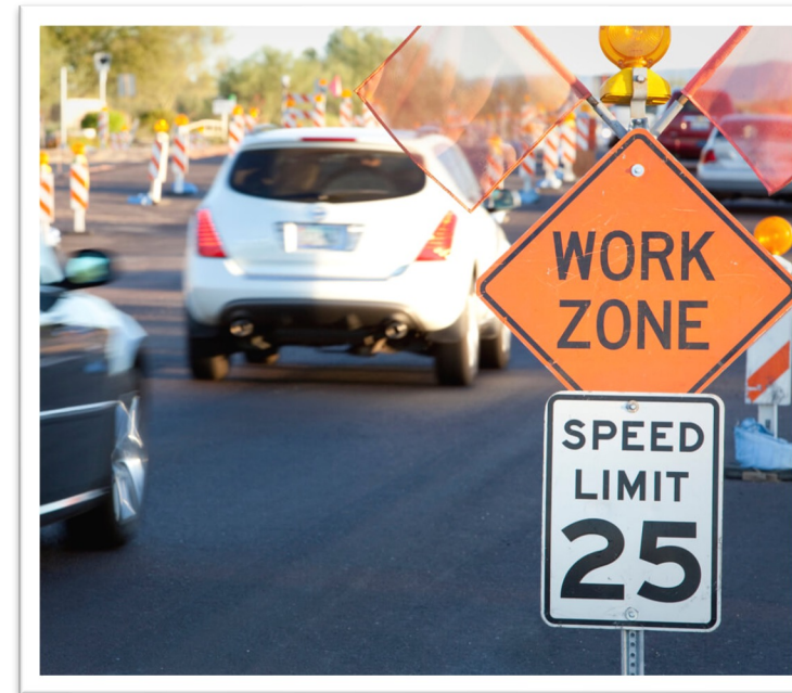
Road Construction and Work Zones
